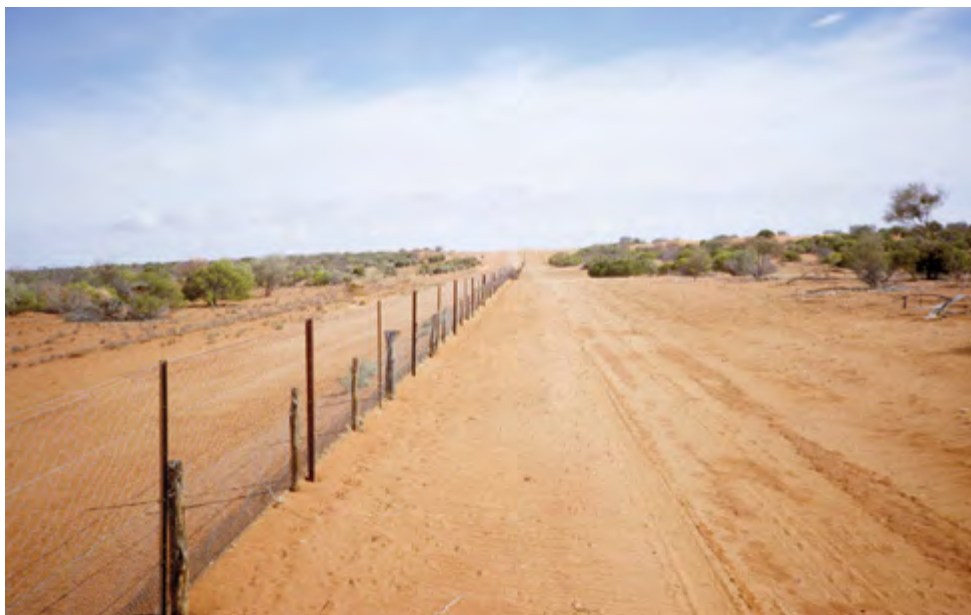
Figure 36. A well constructed and maintained dog fence. (Photo Peter Fleming)
