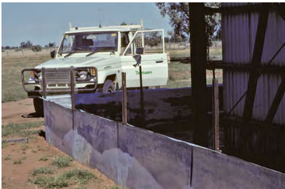
Figure 49. Shed with galvanised barrier. (Photo David Croft)
