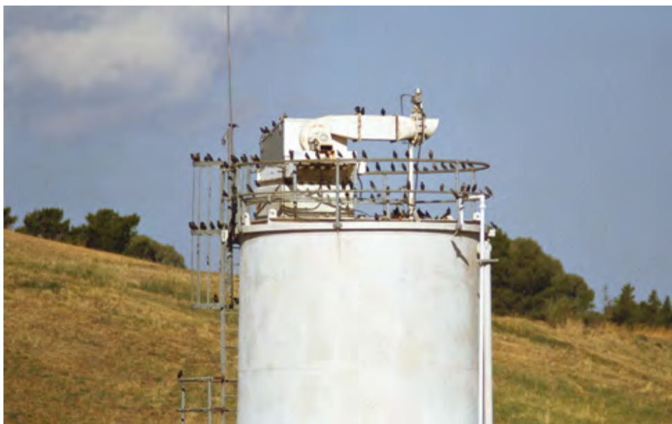
Figure 62. Starlings roosting on a silo. Introduced species such as starlings can defaecate in food storage areas, raising health concerns. (Photo Brian Lukins)
